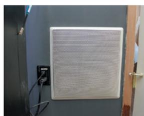
alignment and placement are so important that JL makes three different grille models, with depths to fit wallboards ranging from a half-inch to 19/16 inches thick.
